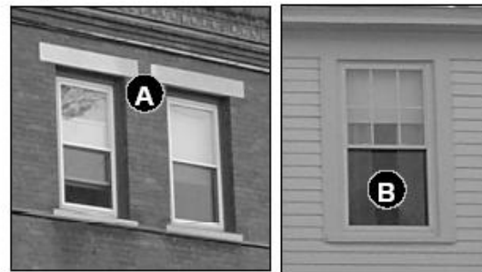
Fig. 25: Examples of proper window treatment. The brick building expresses the structural lintel above the window. Both photos show the storm window is painted and recessed within the window opening.
