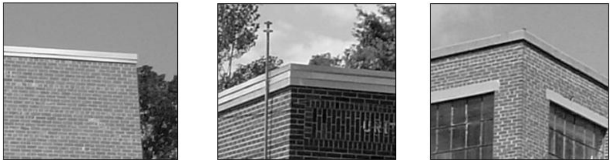
Fig. 8: Unacceptable parapet design. The images above illustrate unacceptable parapet designs for flat roof buildings. These examples show designs which are too thin and lack depth.
