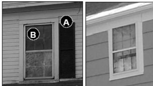
Fig. 24: Examples of improper window treatment. The window on the left has only one (non-functional) shutter, and the storm window is unfinished bare aluminum. The window on the right has a painted storm window, but it is mounted directly to the trim.
