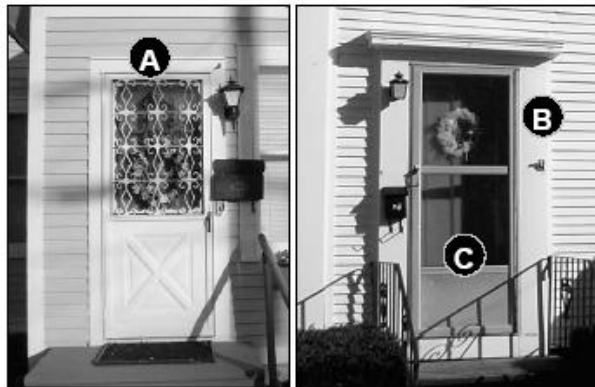
Fig. 22: Examples of improper storm doors. These metal storm doors are mounted on the surface of the wood trim. The white door includes unnecessary detail which does not match the historic design of the house, while the bare aluminum door should be painted.
